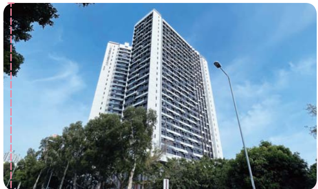
保良局李兆基青年綠洲大樓工程於屆內完成。 The construction of the Po Leung Kuk Lee Shau Kee Youth Oasis was completed within the year.
